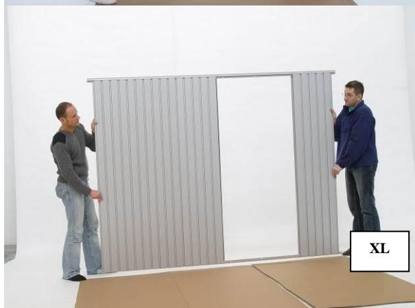
**1. For assembling the side wall** the following parts will be required: the two small front wall panels, the two door posts, one bottom frame profile and the left (right) top profile. To assemble the front wall please consider the advices under point 3.1 to 3.9 of the general assembly manual.
